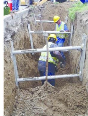
3. Shielding protects workers by using trench boxes or other types of supports to prevent soil cave-ins.
