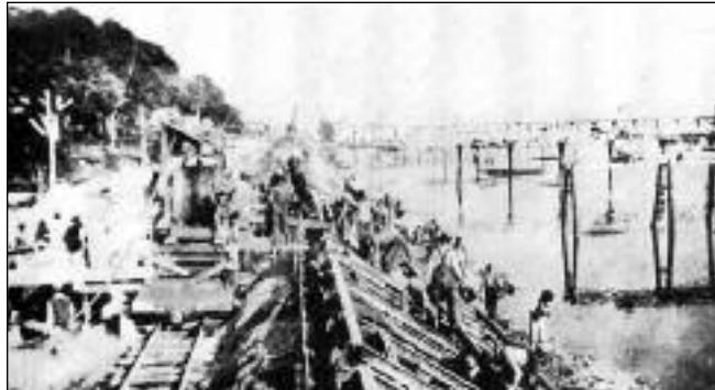
**Figure 3. Construction of the stepped seawall, 1924 (Sullivan, 1985).**
