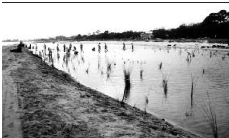
Figure 17. The artificial “cove” constructed as a breakwater during the 2001 renourishment.
