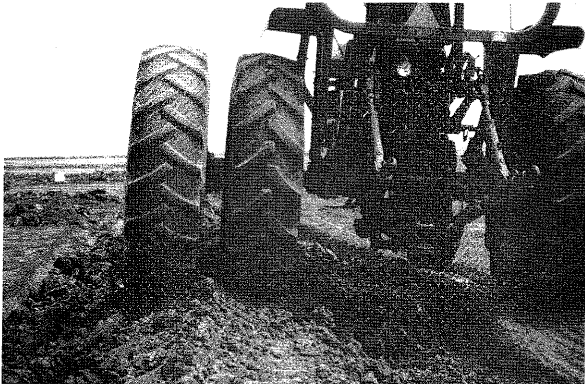
Figure 4. Levee packed with a dual-wheel tractor.
