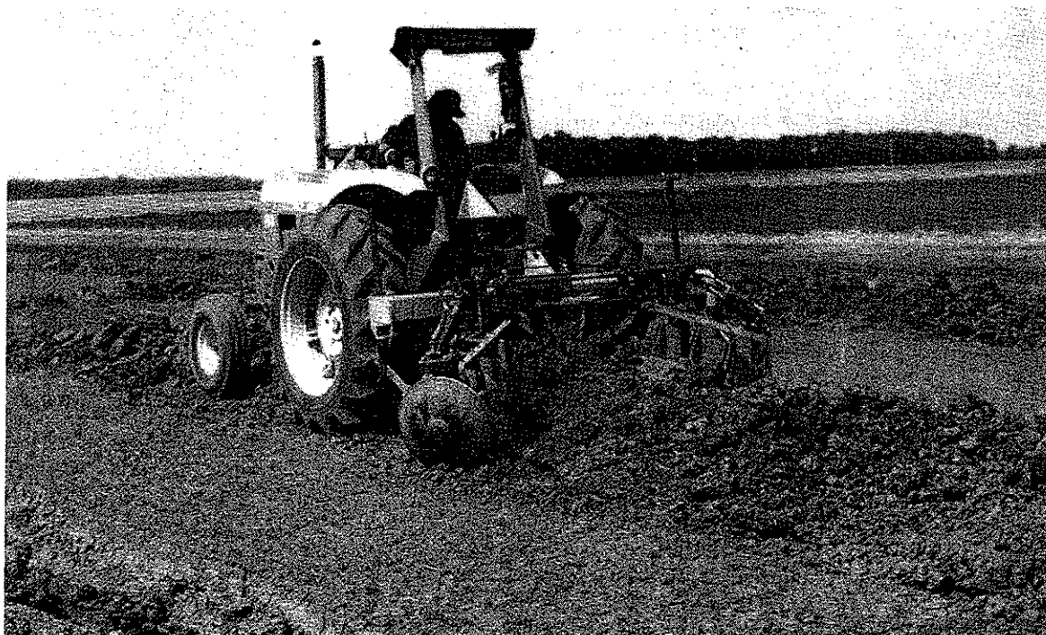
Figure 2. Construction of a basic levee with a levee plow.
