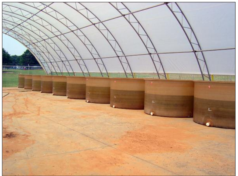
Forty-eight 1,000-gallon tanks will have independent aeration and heating systems.
